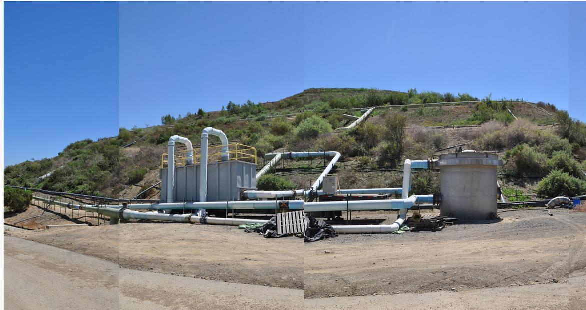
**LANDFILL GAS COLLECTED BY A NETWORK OF PIPES FUELS TWO GAS-TO-ENERGY PLANTS. ELECTRICITY PRODUCED POWERS 70,000 HOMES, THE SAN JOSE CREEK WATER RECLAMATION PLANT AND SANITATION DISTRICTS OFFICES.**
