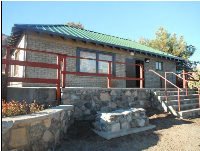
Figure 6. Northern Facade of DPB-001 (view southwest; October 19, 2022).
