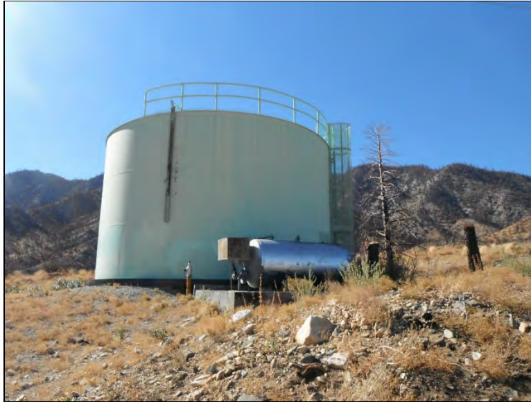
Figure 9. Northern Side of DPB-003 (view south; October 19, 2022).
