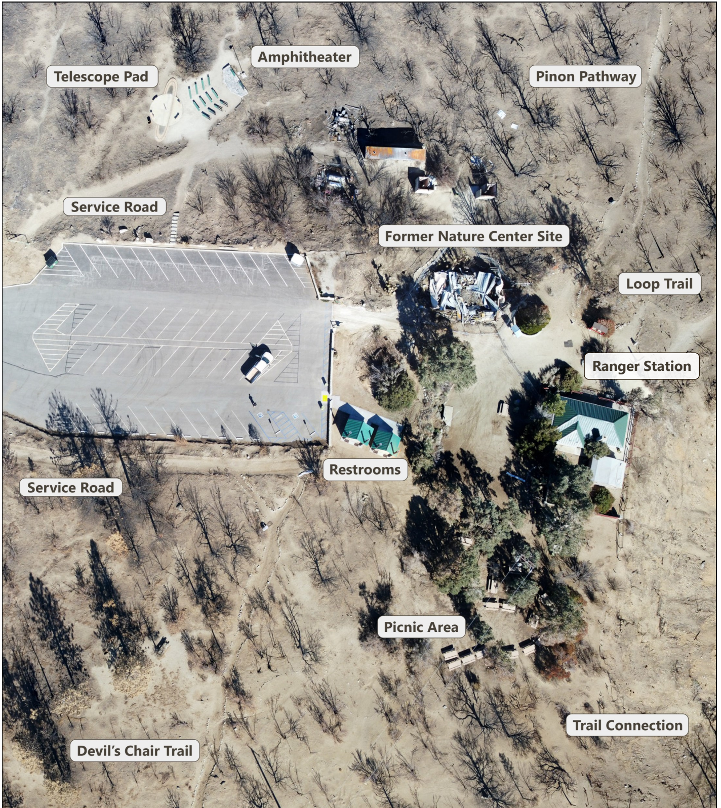
Figure 3. (Above) depicts the extent of structural damage at the Devil's Punchbowl Natural Area after the 2020 Bobcat fire. In addition to the newly installed restroom facilities, the remaining healthy trees, existing parking lot, picnic area, trailheads, telescope pad and amphitheater are to remain in place.
