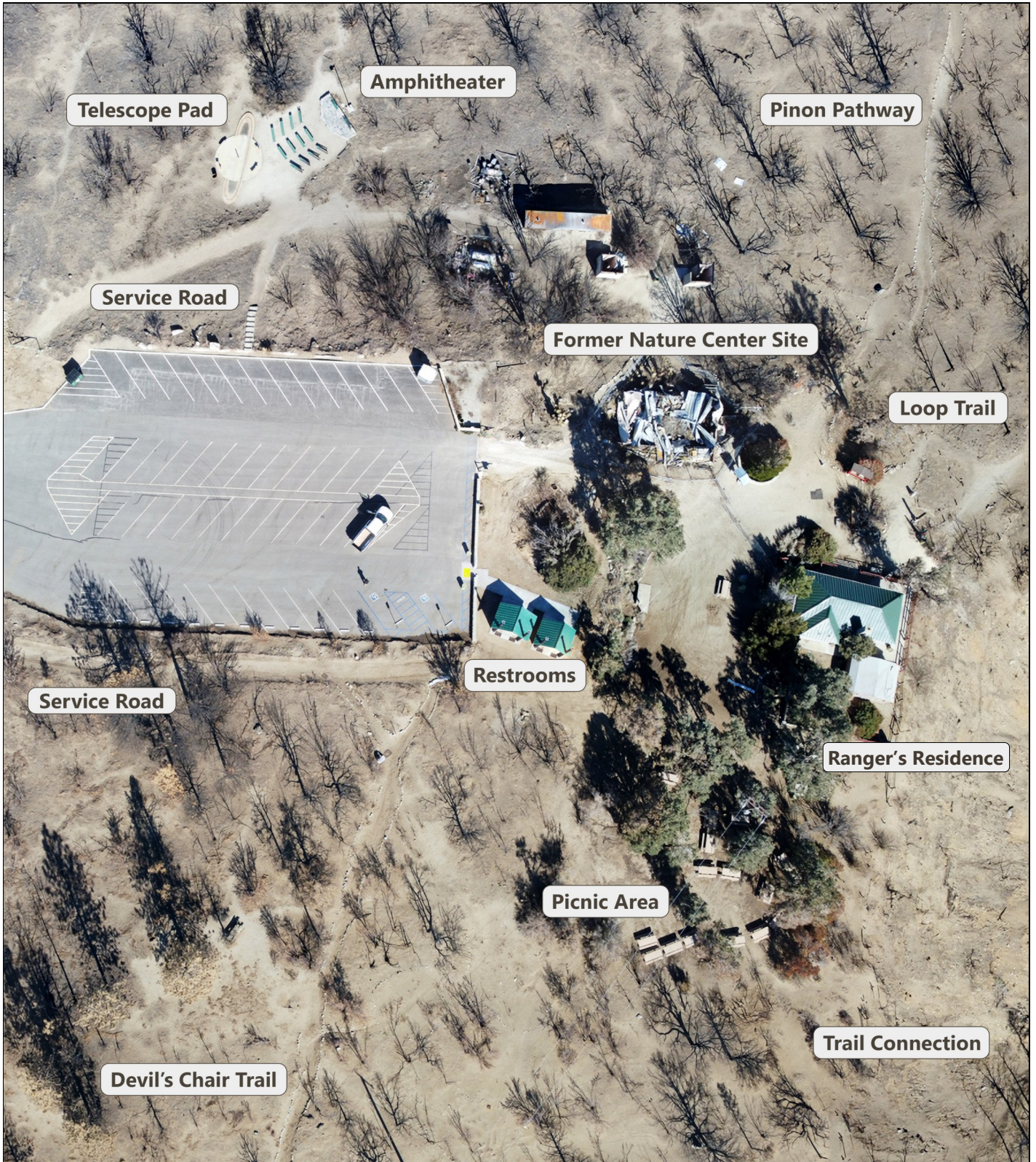
Figure 1-1 (Above) depicts the extent of structural damage at the Devil's Punchbowl Natural Area after the 2020 Bobcat Fire. In addition to the newly installed restroom facilities, the remaining healthy trees, existing parking lot, picnic area, trailheads, telescope pad and amphitheater are to remain in place.
