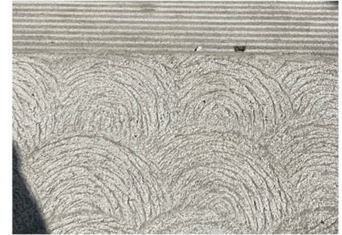
Rough Textured Concrete At Shared Tread Concrete Underpasses
