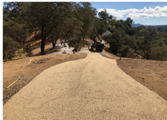
Chip Seal Paving
